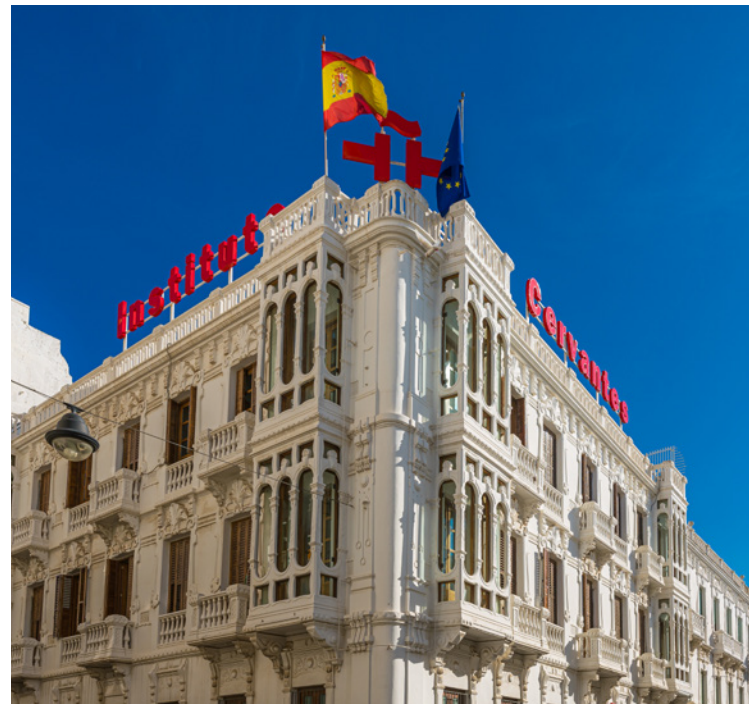
Facade of the headquarters of Instituto Cervantes in Tétouan, Morocco.
